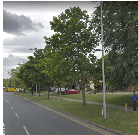
Fig 8.2 Existing DLRCOCO Public Lighting columns on Carmanhall road
